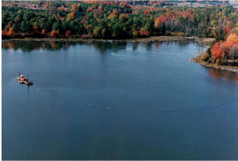
Figure 11. Hydraulic Dredging Barge
