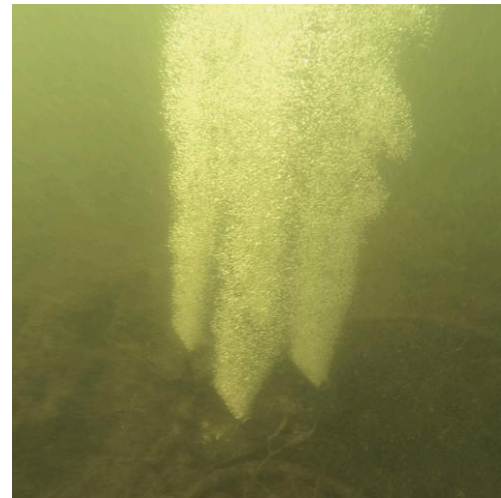
Aerator on lake bottom.
