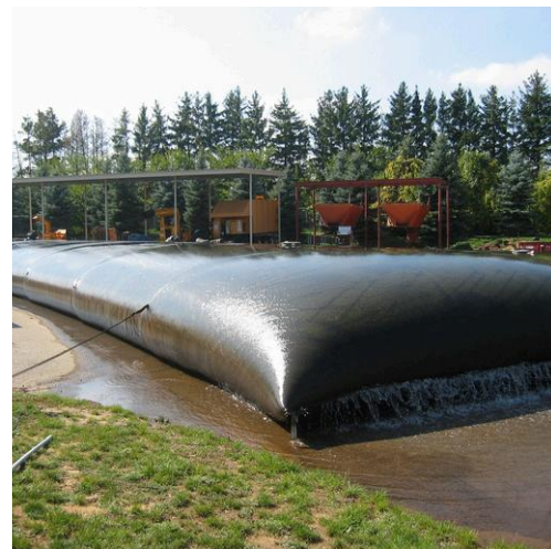
Hydraulic dredging geotextile dewatering bag.
